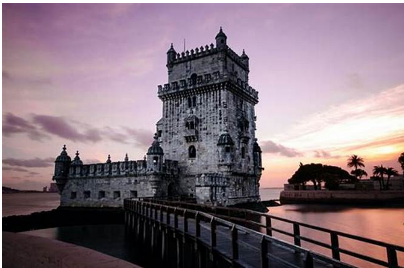
The Tower of Belém in Lisbon
